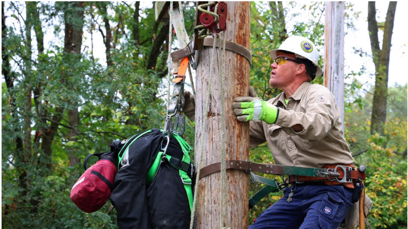
Village lineman Lane Dykman at the recent AMP rescue training.
